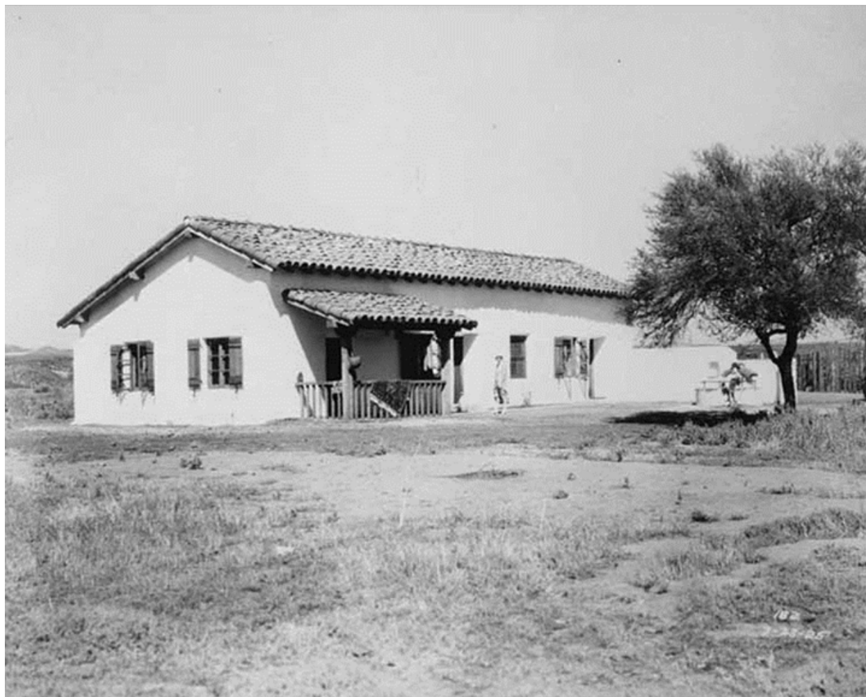
Figure 10. Juan María Osuna Adobe looking northeast, circa 1925. The photo shows the completed Lilian Rice rehabilitation. New tile roofing, plaster, windows, wood shutters, doors, railing, and front porch have been added. Source: Rancho Santa Fe Historical Society.
