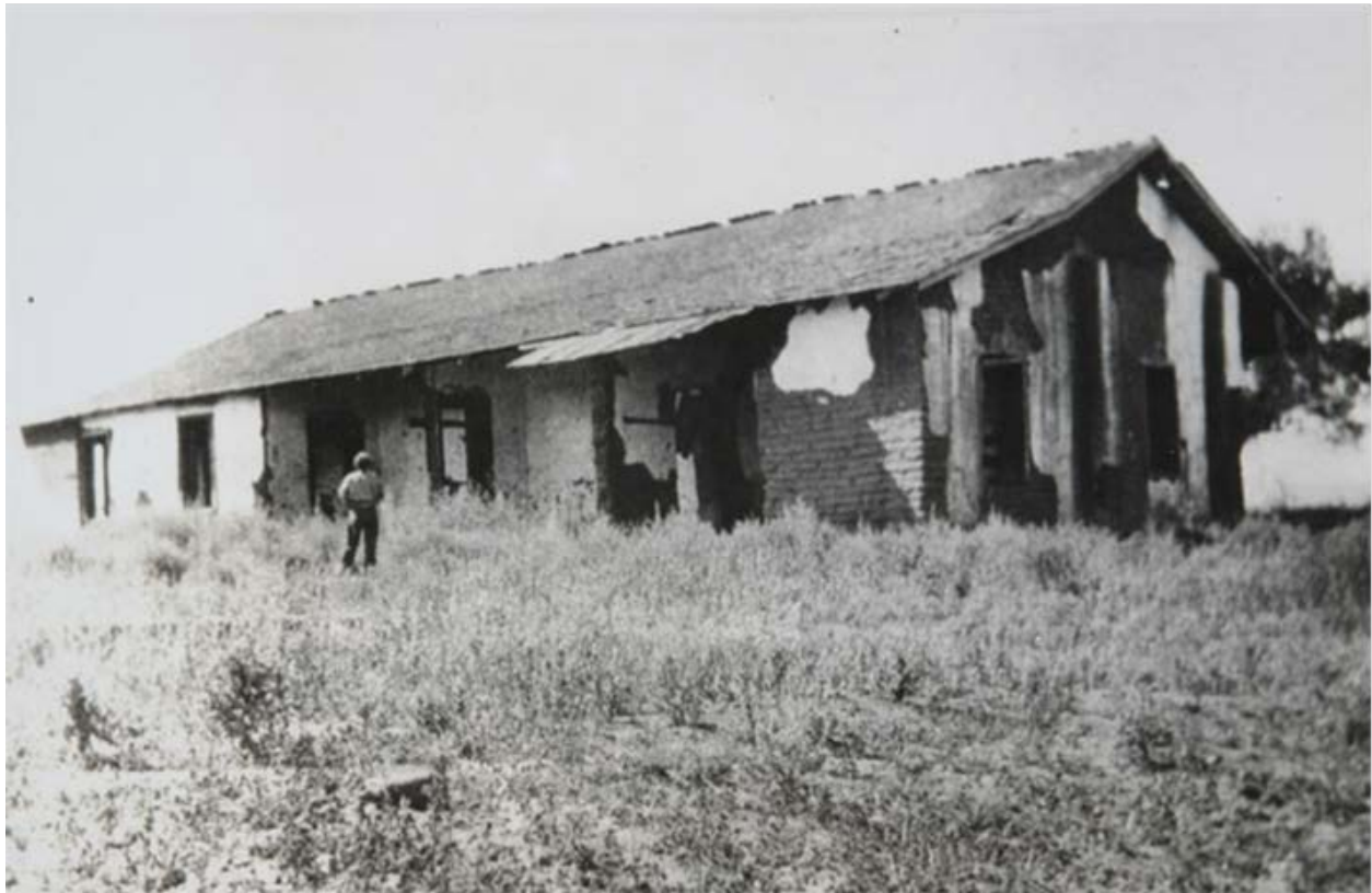
Figure 5. Juan María Osuna Adobe, circa 1920, prior to the Lilian Rice rehabilitation, looking south. The photo shows a wood shingle roof and no chimney. The wall finish appears to be mud plaster with whitewash. Source: Southwest Museum.
