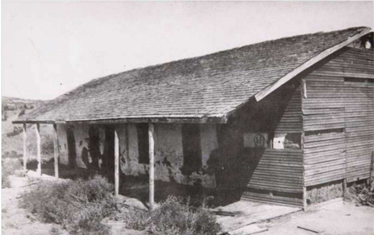
Figure 7. South elevation showing the original porch that extended along the entire south elevation with a raised wood porch deck. Source: Southwest Museum.
