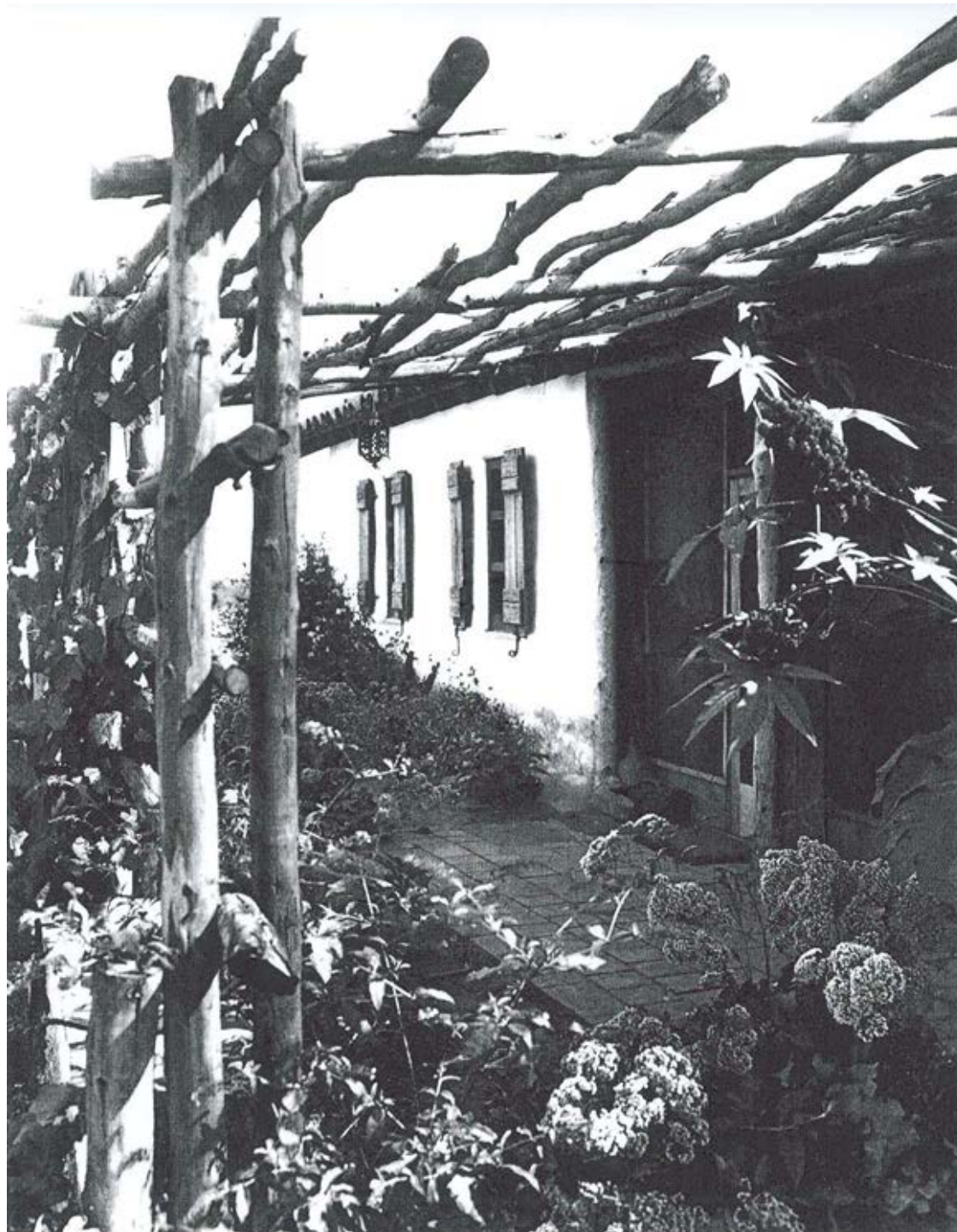
Figure 15. The rear porch shows the historic porch with a rustic wood trellis. The historic porch flooring is scored concrete matching the sleeping porch, circa 1925. Source: Rancho Santa Fe Historical Society.
